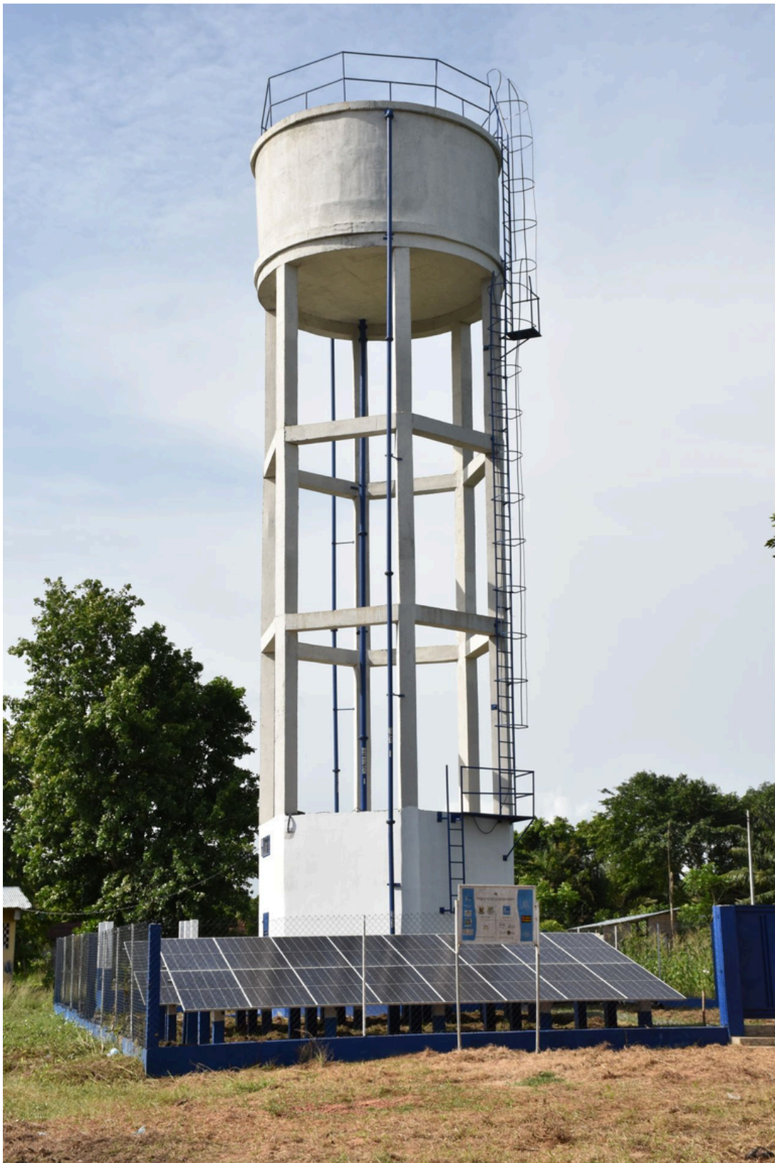
Water tower Bas-Mono, Togo
